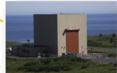
Payload Processing Facility
