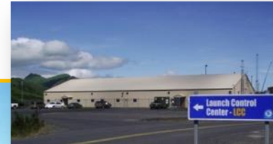
Range Control Center
