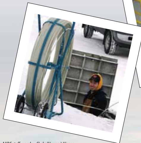
AADC staff member Clyde (Hopper) Hinson lays fiber optic cable. AADC Archive Photo
