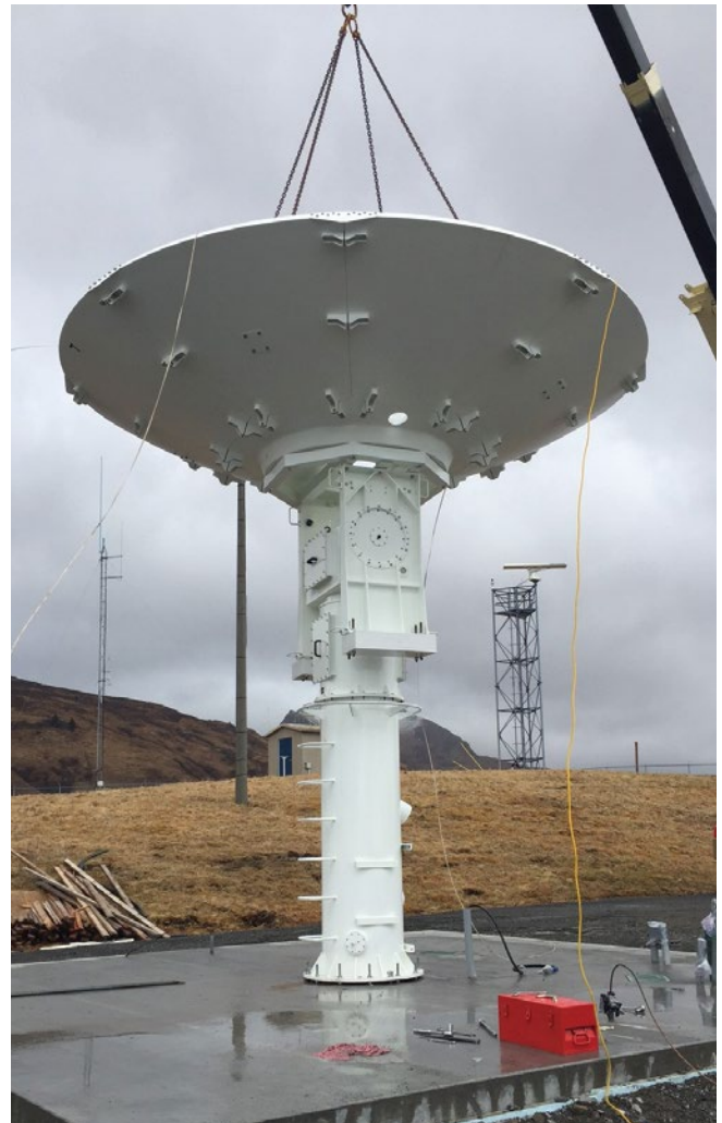
New telemetry antenna installation at PSCA.
