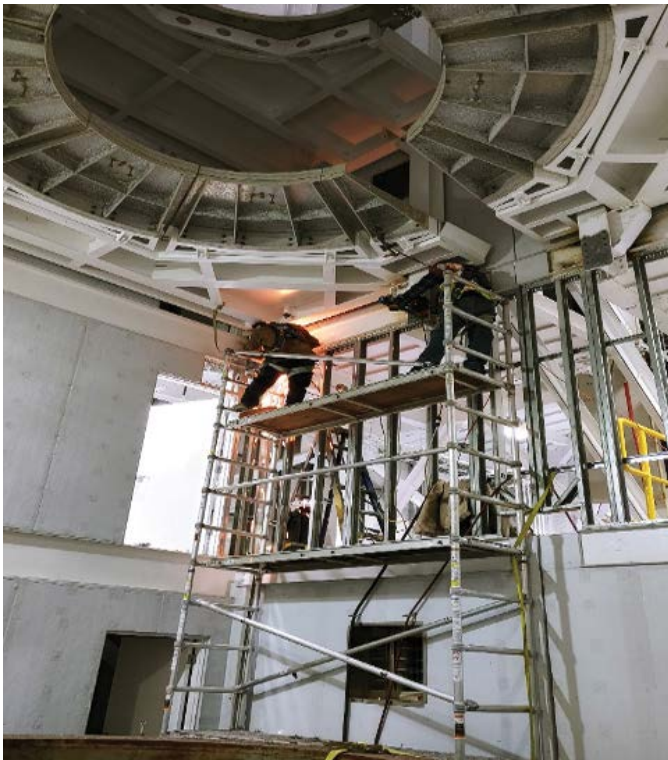
Building of the Tower for thermal insulation.
